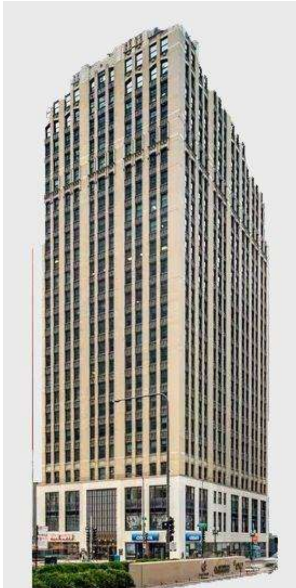
Chicago's First Network Radio studios NBC, Lake Michigan Building
