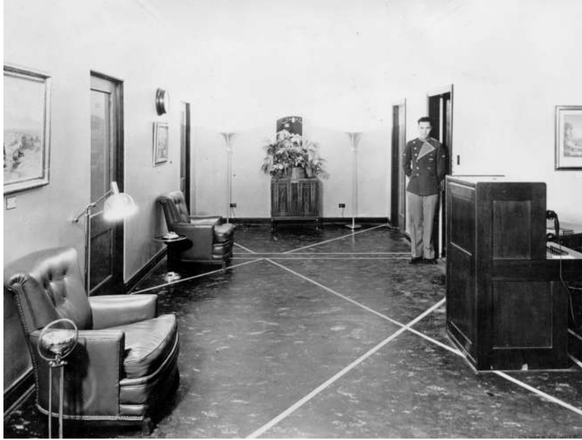
Main Reception area—fourth floor.
