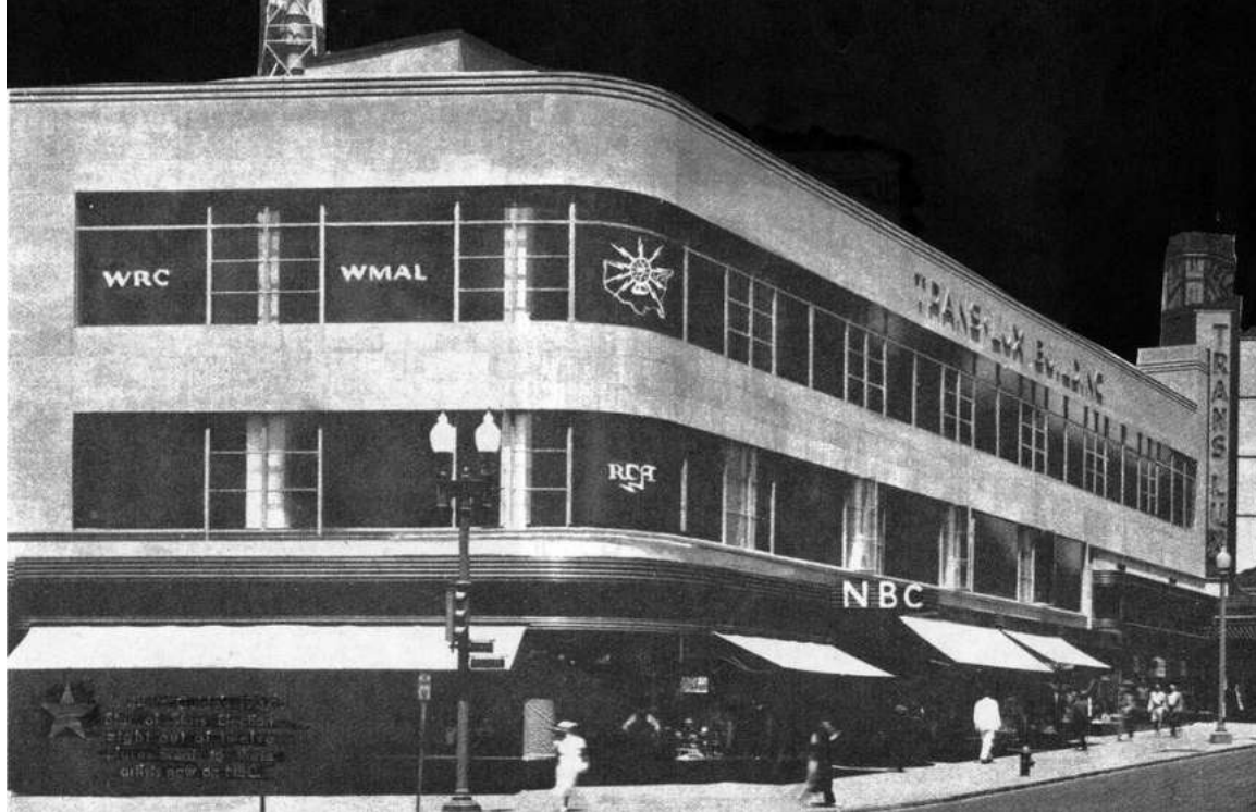
Built on a slope, the Trans-Lux building had three floors at one end sloping toward the theatre area which intruded into a portion of the second floor.. RCA leased the majority of the second floor and NBC and WMAL occupied the entire third floor. [Courtesy of the Library of Congress]
